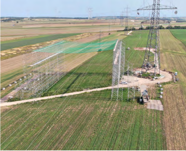
The new Weinviertel line comprises 202 pylons, each of which is around 60 metres high.
