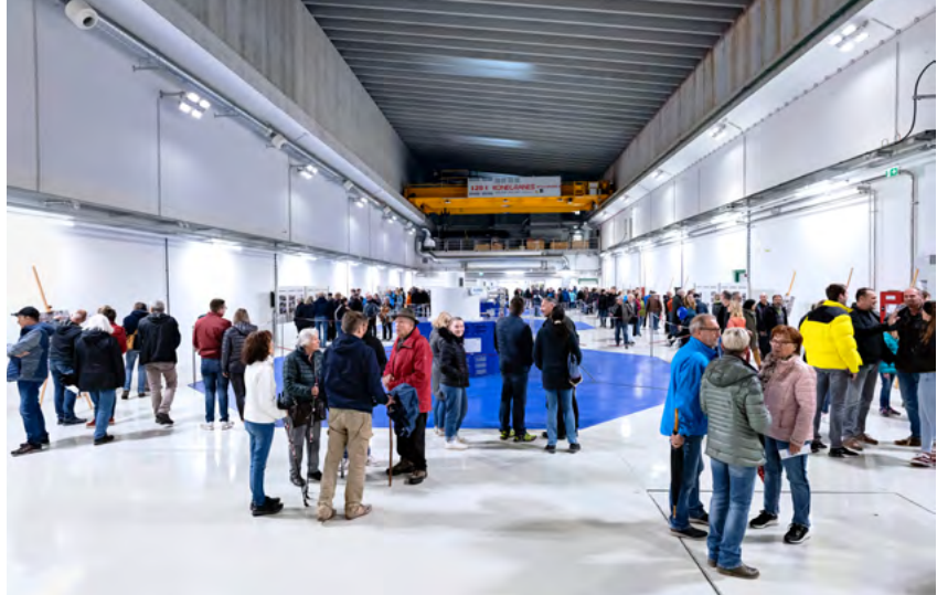
Well-attended: the Open Day held at the new Töging powerhouse on 1 October 2022 gave the many visitors the opportunity to form their own impression of the project.
