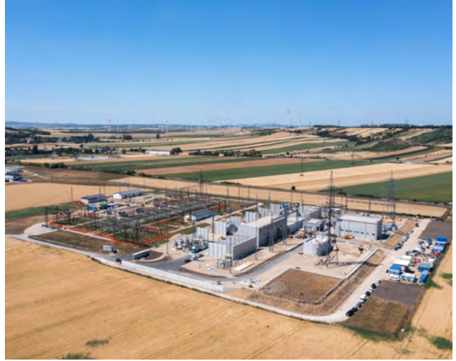
A new substation in Neusiedl an der Zaya was also built as part of the project.
