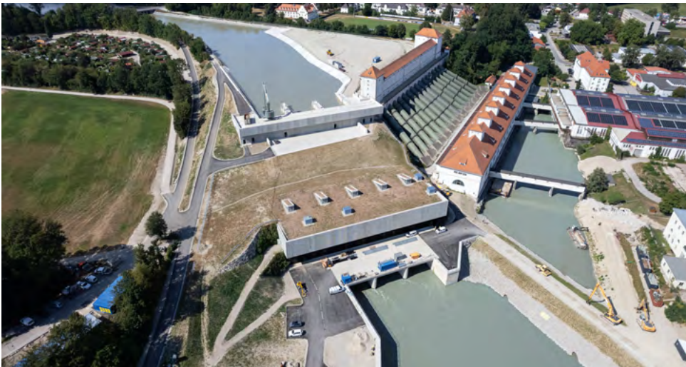
Töging hydropower plant: the new building for the Töging powerhouse (centre) with the existing installation in the background on the right (8 August 2022)
