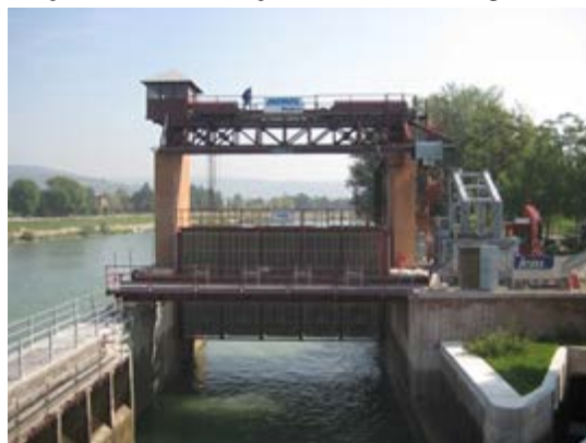
Figure 5-3: Abandoned canal locks from the 19th century, equipped with five innovative generating modules with a capacity totalling 1.35 MW without compromising its discharge capability.
