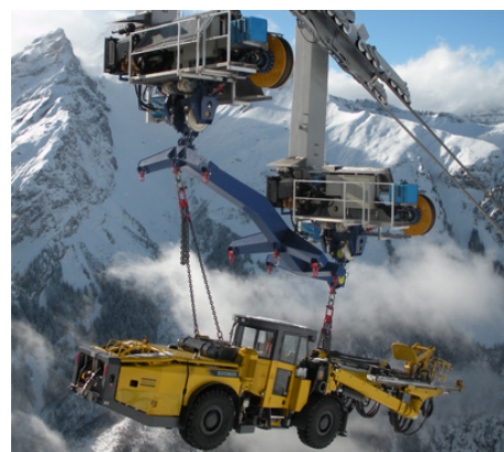
Figure 5-6: Largest cable lift systems in the world, installed for the pump storage power plant project 'Linthal 2015', Switzerland Source: www.freyag-stans.ch
