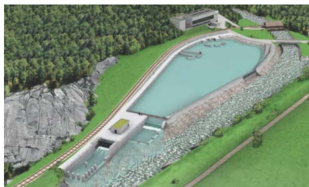
Figure 5-4: Compensation basin to reduce hydropower-peaking at power plant Innertkirchen, Switzerland
