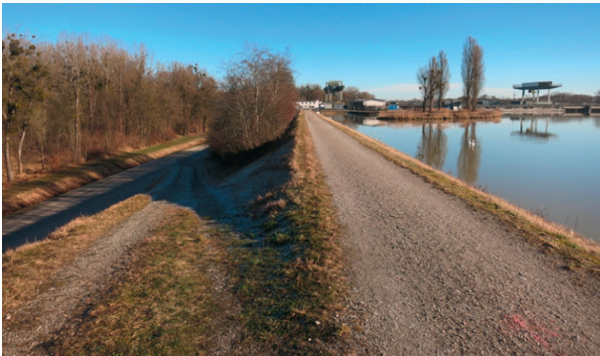
Project region in the head pond of the Ering-Frauenstein power plant
