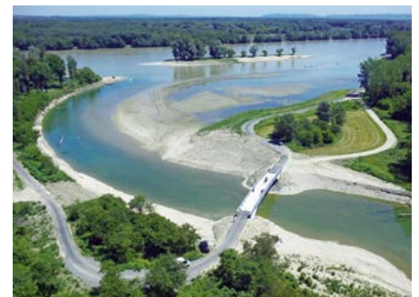
Project to restore the estuary stretch of the Traisen River in Lower Austria
