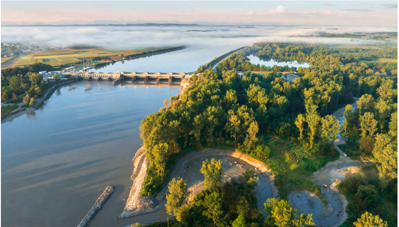
View from the tailwater area on the Braunau-Simbach hydropower plant
