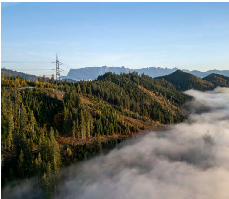
The new 380-kV Salzburg line will enable efficient integration of renewable energies into the Austrian power grid.
