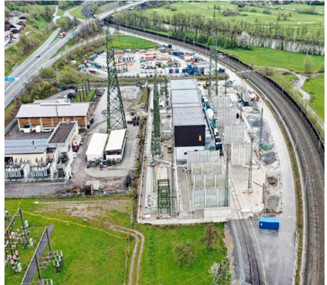
The project also involved building a new substation in Pongau.
